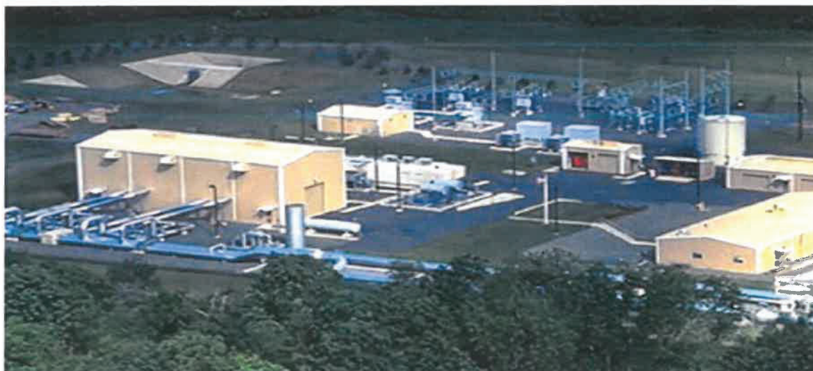
Gas transmission compressor station.
