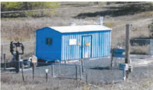
City gate meter station.
