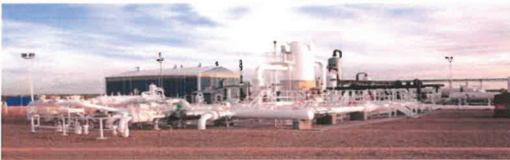
Natural gas compressor station.
