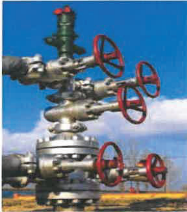
Natural gas wellhead.
