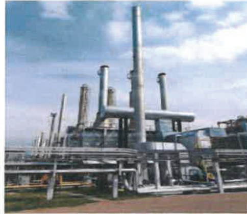
Natural gas processing facility.
